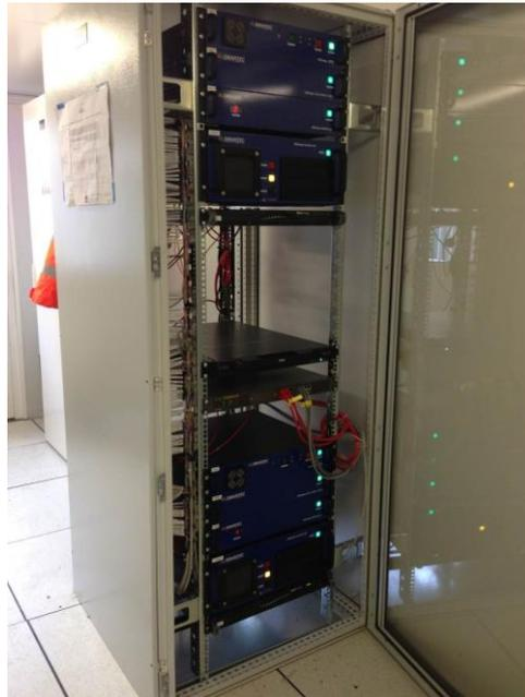
**Fig. 9: Implementation of a leakage detection system, including fully redundant DTS, multiplexer, realy module, ATTS and processing PC**
