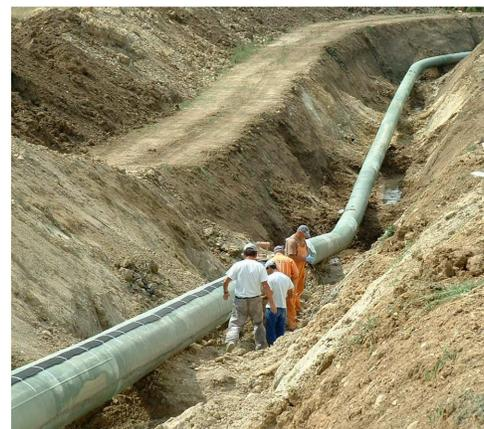
Fig. 6. SMARTape installed on the gas pipeline.
