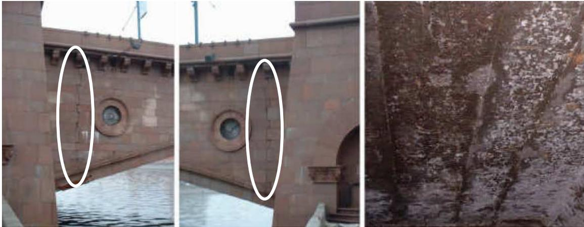
Fig. 3. Cracking of the stone walls (ellipses on left photos) confirms the settlement in the middle of the arch; penetration of chlorides is visible in the interior of the arch boxes (right photo).
