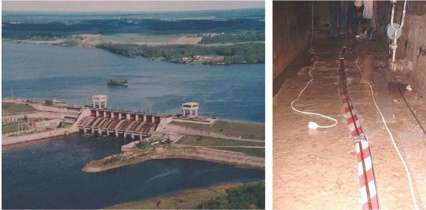
Fig. 5. General view of Plavinu dam in Latvia (left) and SMARTape installation in the inspection gallery (right).
