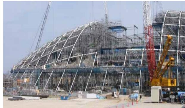
Fig. 20. Dome Jack-up construction stage
