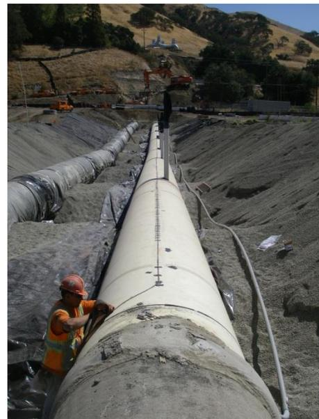
Figure 10: Water pipeline section crossing tectonic fault and instrumented with distributed strain sensors (visible on top, two other lines installed at 4 and 8 o'clock).
