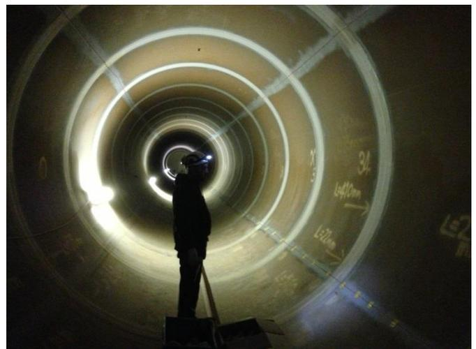
Figure 11: Penstock equipped with four lines of longitudinal strain sensing cables. The white circumferential strips are the sealing rubber bands.
