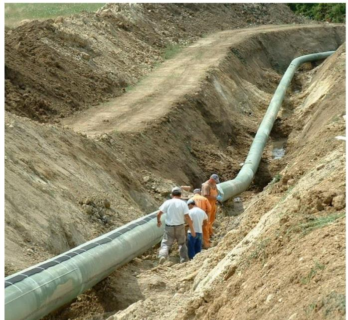
Figure 7: SMARTape on the gas pipeline.
