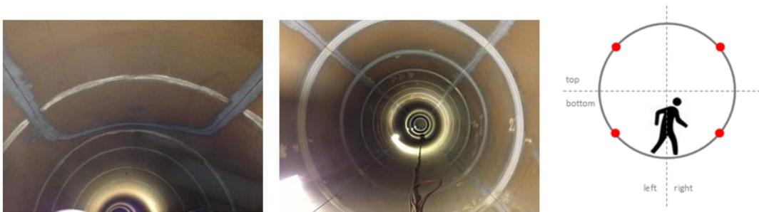
Figure 10 SMARTprofile sensor installation inside the penstock.
