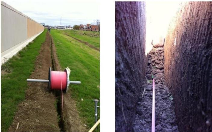
Figure 5. Installation of SMARTprofile sensor in a trench on the surrounding of the levee wall.
