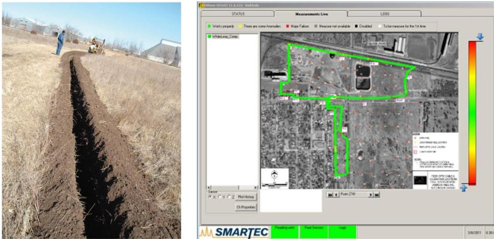
Figure 8 Installation of Reinforced Hydro & Geo sensor in a trench and cable path on map.
