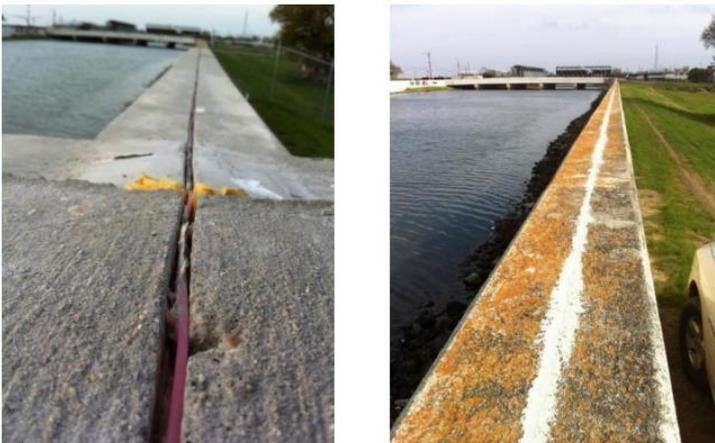
Figure 6. Installation of SMARTprofile sensor in a groove on top of the levee wall section.
