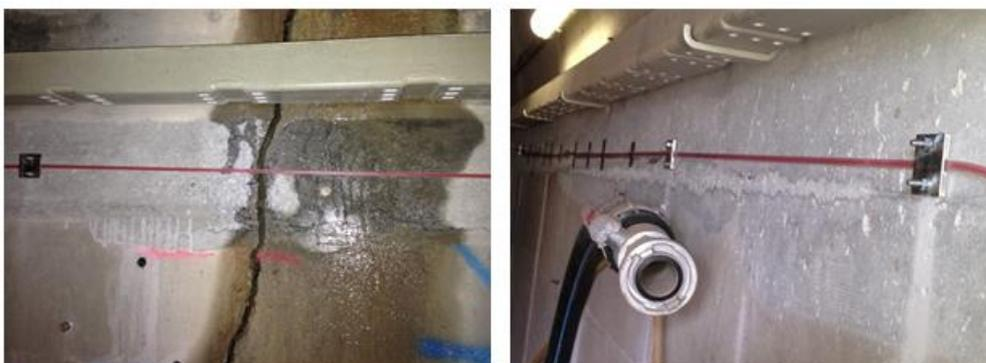
Figure 11 SMARTprofile sensor installation on penstock access tunnel.
