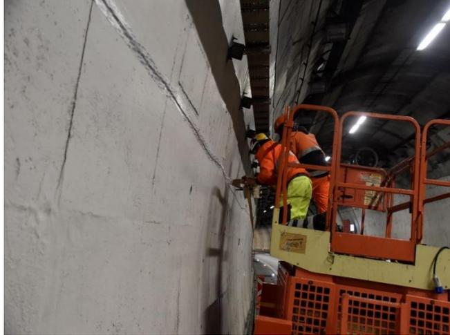
Figure 4. SMARTProfile sensor installation on the tunnel lining.
