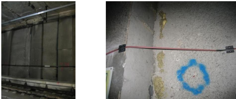
Figure 6. Sensor installation in the high-speed rail tunnel in Spain.
