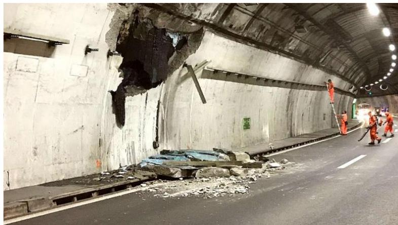
Figure 3. Local collapse of the San Salvatore Tunnel vault.
