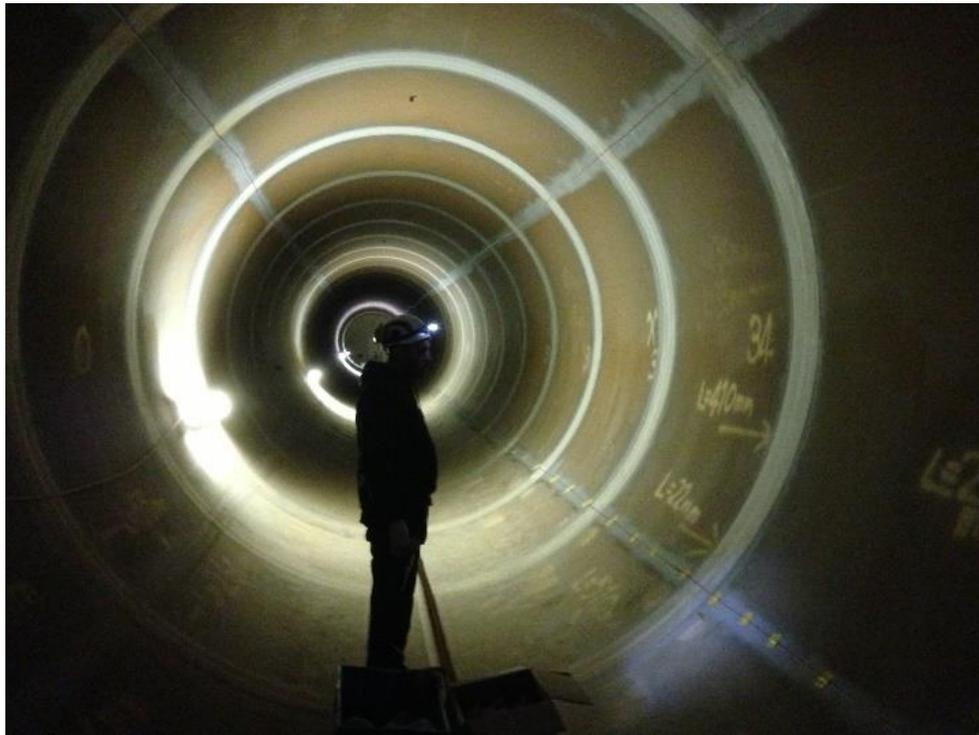
Figure 7. Penstock equipped with four lines of longitudinal strain sensing cables. The white circumferential strips are the sealing rubber bands.
