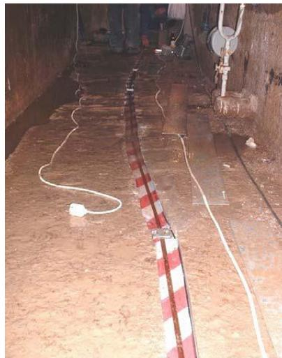
*Figure 14: Installation of SmarTape and Temperature Sensing Cable*
