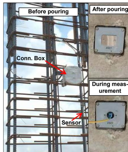
Figure 4. Sensor and connection box installed on a rebar cage, and connection box after the pouring of columns
