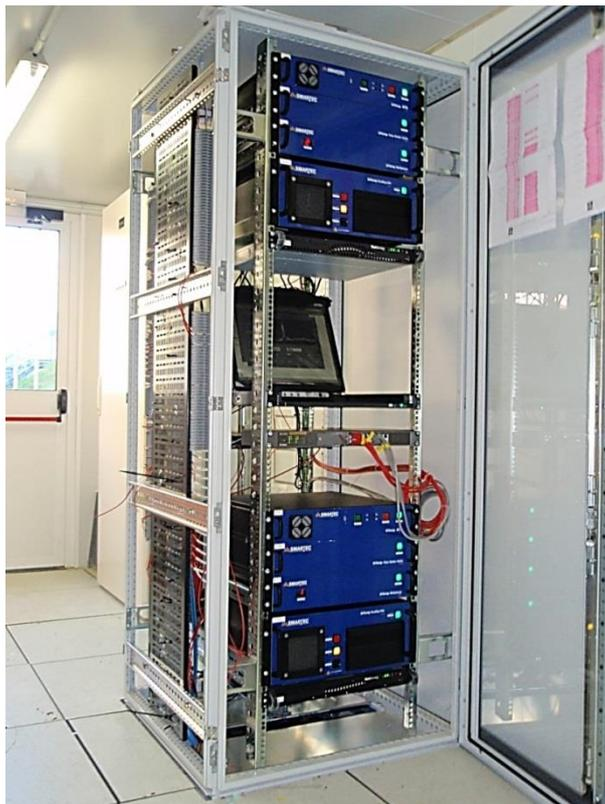
Fig. 1: Fully redundant leak detection system
