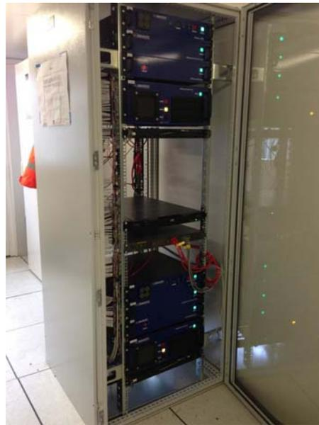
Figure 9. Implementation of a leakage detection system, including fully redundant, DTS, Multiplexer, Relay module, ATTS and processing PC
